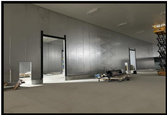
Production Room Entrance
